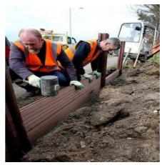
3 foot of water and protect up to 30 properties from flooding in the future. It was confirmed that the scheme was one of several to receive funding from the EA. The photograph above shows the erection of the flood wall at Waldridge.
